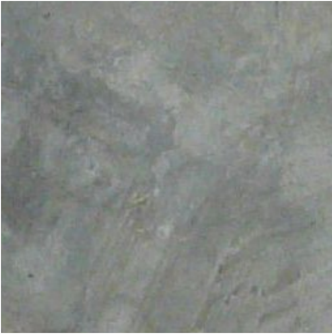
Polished and stained concrete flooring downstairs
